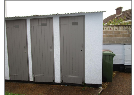
2 Exterior Storage Sheds
